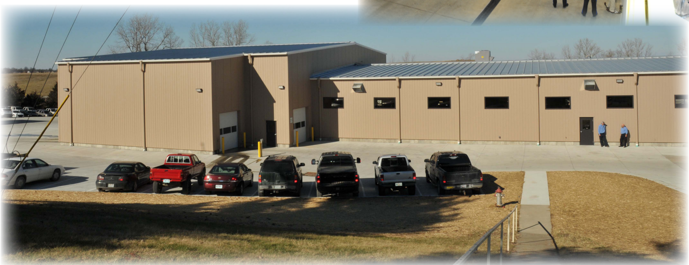
This state-of-the-art facility opened February 4, 2016, replacing the old GHQ Garage which was destroyed by fire.
