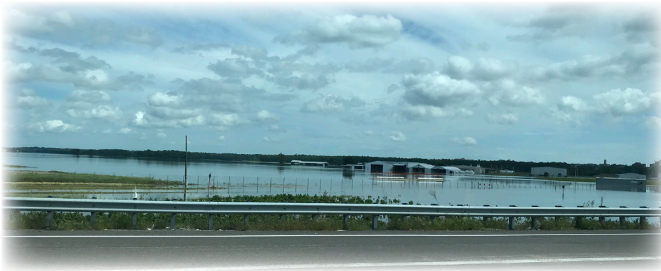
The Jefferson City Airport closed for weeks due to flooding.
